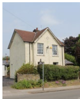
Left: Bay windows, hip roofs and front-projecting gables.
