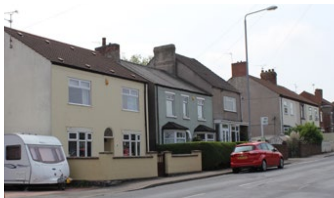
Left: Buildings placed hard against the back edge of the footpath.
