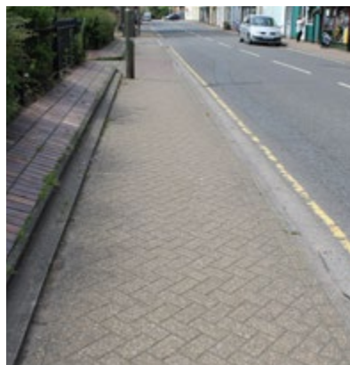
Left: Dead frontages to the street on the old Co-op store.
