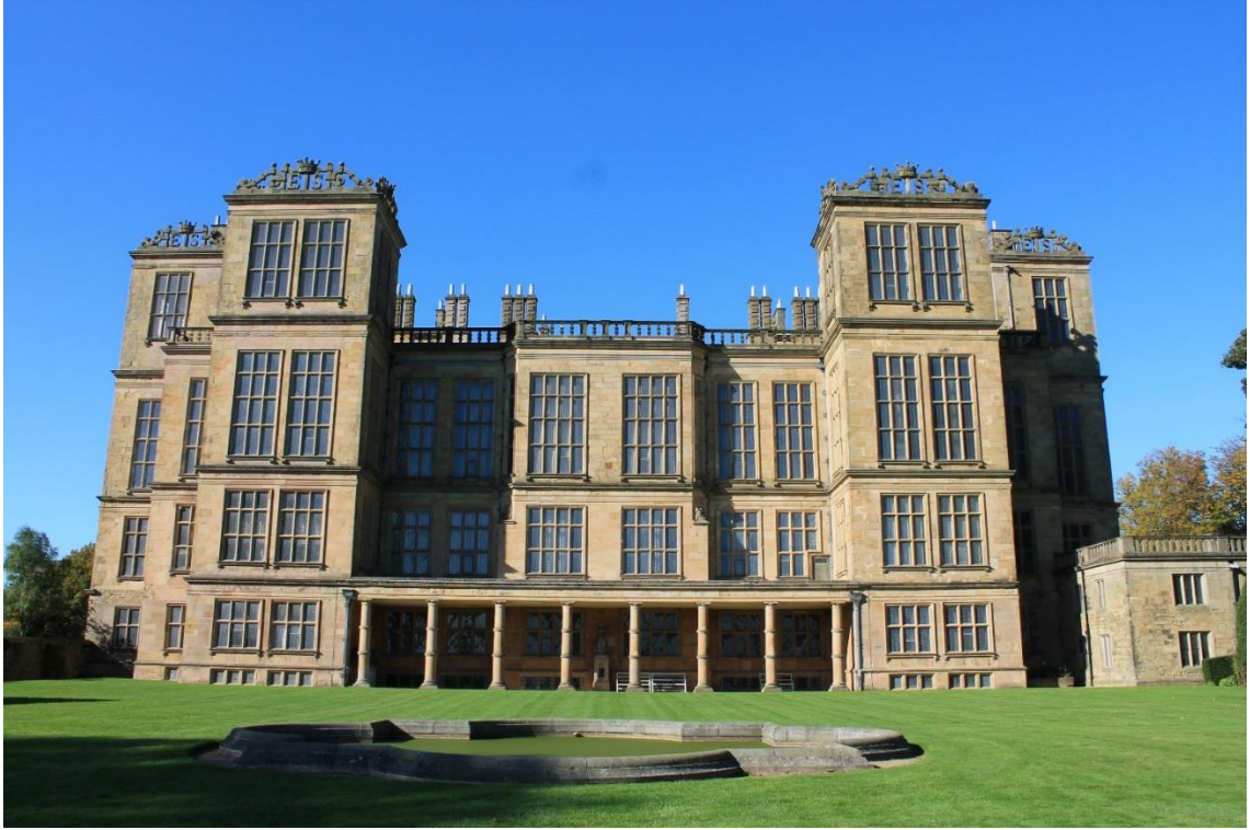
Figure 3. The East Façade of Hardwick Hall
