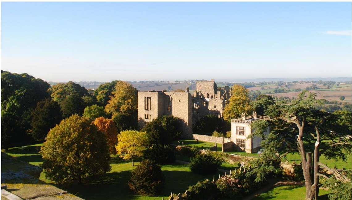
Figure 1. The 'disorganised' Old Hall, pictured from the roof of the New Hall
